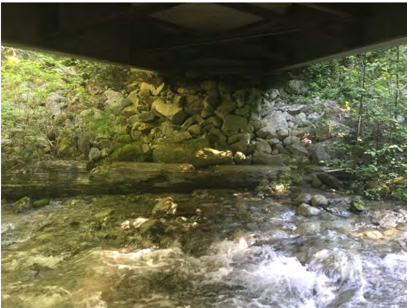
Right Bank Abutment when facing downstream
