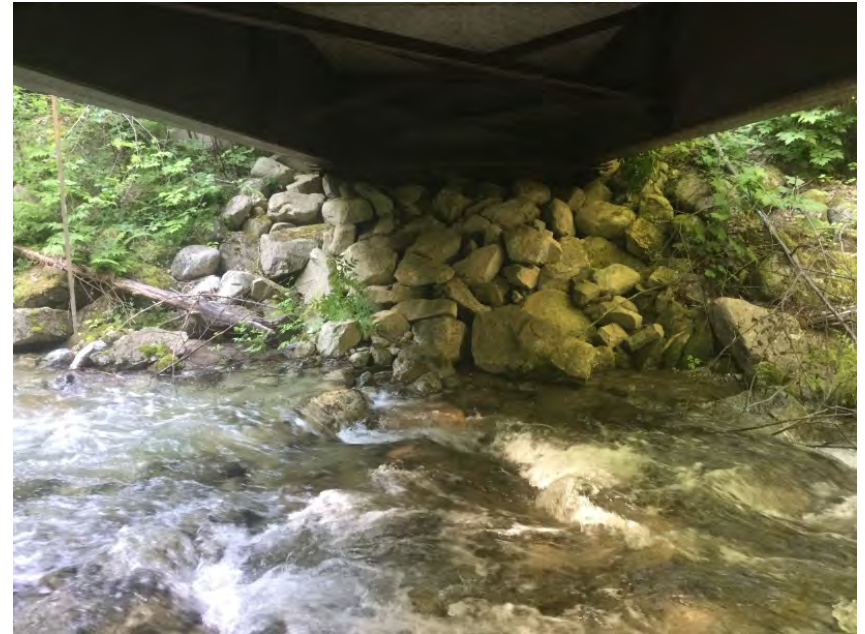
Left Bank Abutment when facing downstream
